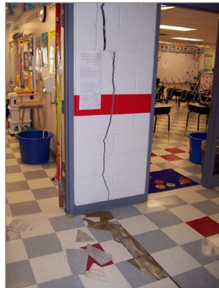
The Benld Elementary School sustained irreparable damage as a result of mine subsidence on March 27, 2009.
