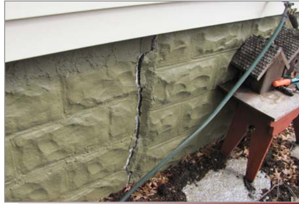
On April 8, 2015 approximately 15 homes in Benld sustained foundation damage as the result of mine subsidence.
