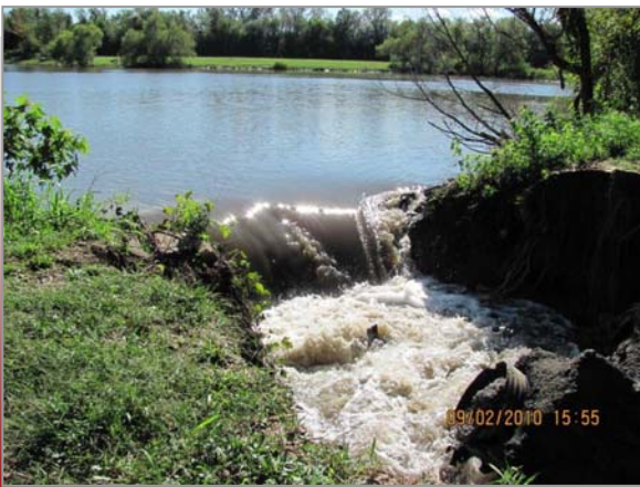
The Virden Recreation Club Lake Dam suffered a catastrophic dam failure on September 2, 2010 that resulted in the conversion of the Lake back to farmland.
